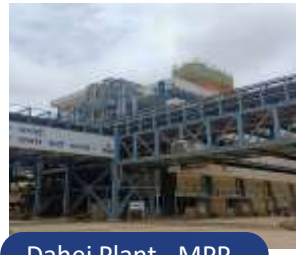
Dahej Plant - MPP
