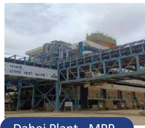
Dahej Plant - MPP
